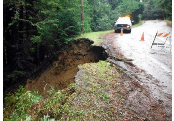
One example of storm damage is along Palo Colorado Road in Big Sur. Floodwaters in Rocky Creek caused the culvert under the road to fail (below) and major road damage (above). Palo Colorado Road is closed here, with only foot traffic allowed until repairs can be made.
