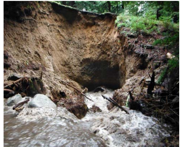
One example of storm damage is along Palo Colorado Road in Big Sur. Floodwaters in Rocky Creek caused the culvert under the road to fail (below) and major road damage (above). Palo Colorado Road is closed here, with only foot traffic allowed until repairs can be made.
